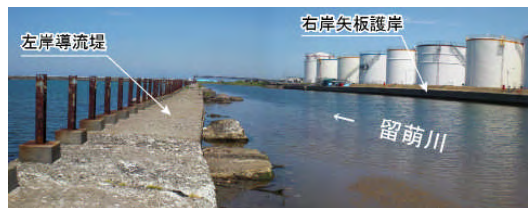
図-3 既設導流堤・護岸の状況
